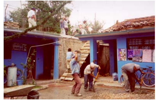
Theater under construction Photograph courtesy of Christine Eber
